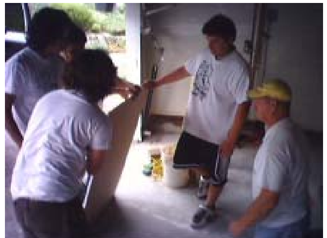
Ron Rhodes and student workers take a measurement on the sheetrock.
